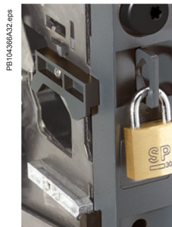
"Disconnected" position locking by padlocks.
